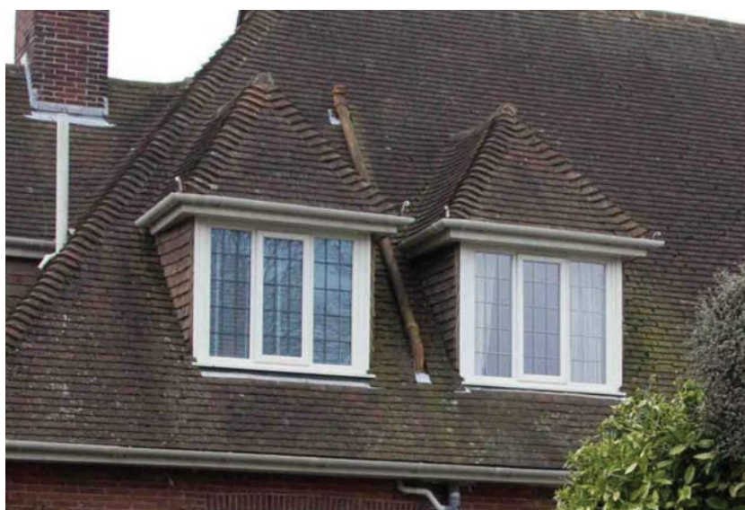
Picture 20 Original dormer windows.
