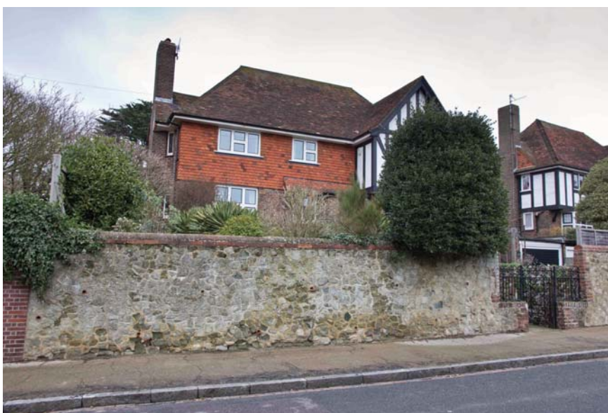
Picture 14 No. 3 Torfield Road, clay tile hangings and timber frame to gable.
