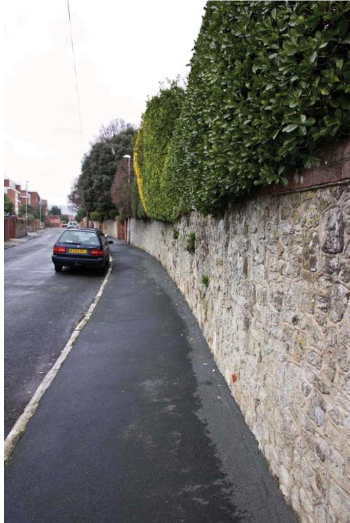
Picture 2 Selwyn Road, boundary walls.
