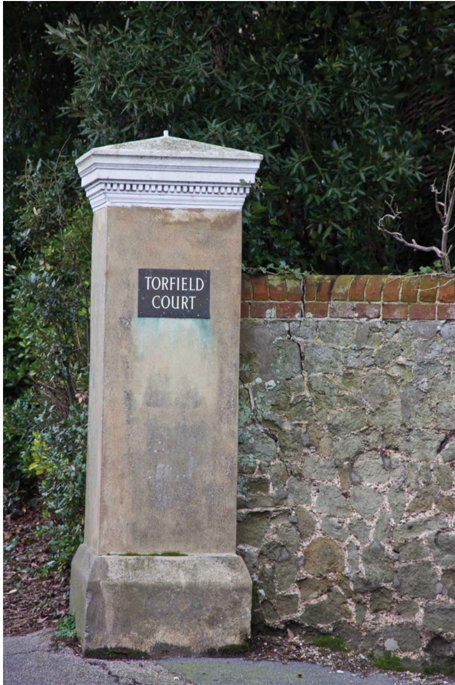
Picture 5 Torfield Court pier, St Anne's Road.
