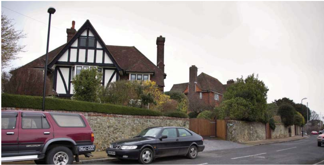
Picture 16 No. 1 Tor Hay, note the tall chimneystacks and hipped clay tile roof.
