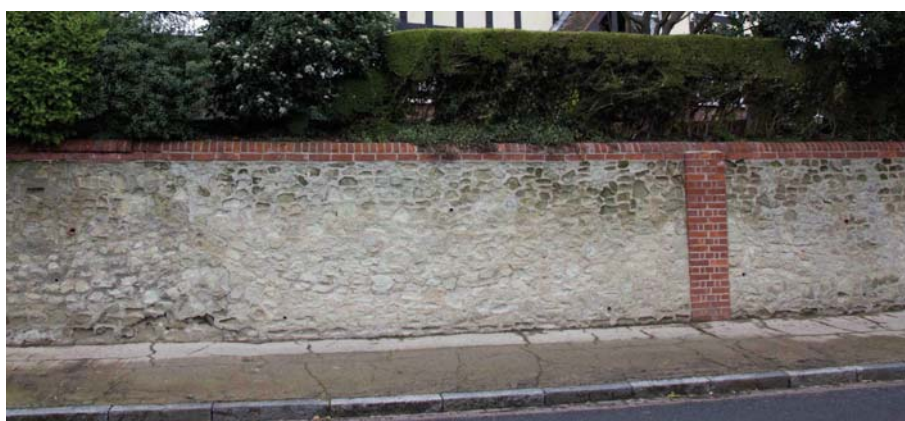
Picture 21 Example of original boundary walls.
