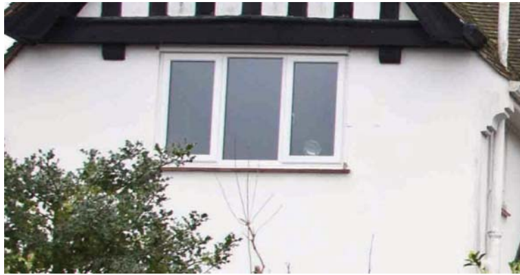
Picture 19 UPVC replacement windows.
